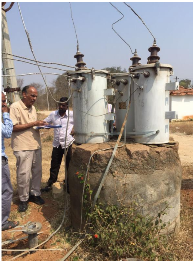
Satish Chaparala inspects improperly installed power distribution transformers a common problem in the rural area of Hyderabad India.
